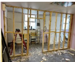
Renovation at church for kids club ministry.
